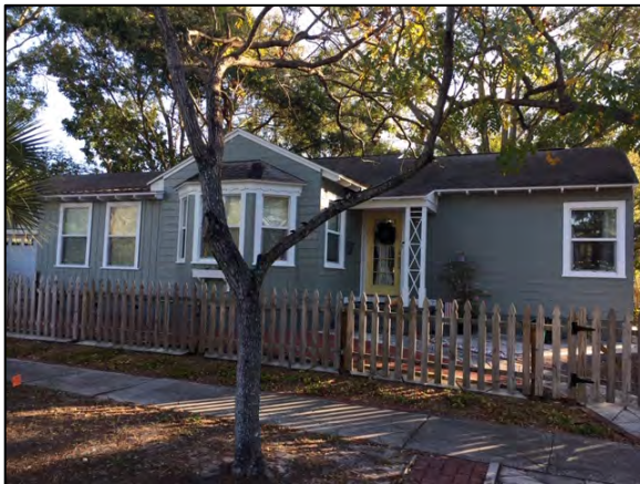
Figure 6: Three-foot wooden front and side yard fence with high transparency in subject district (3163 6 th Ave. N.)
